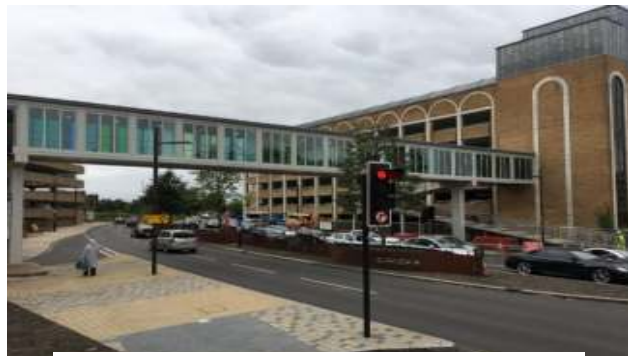
Figure 3.3: Queensgate Footbridge Refurbishment
